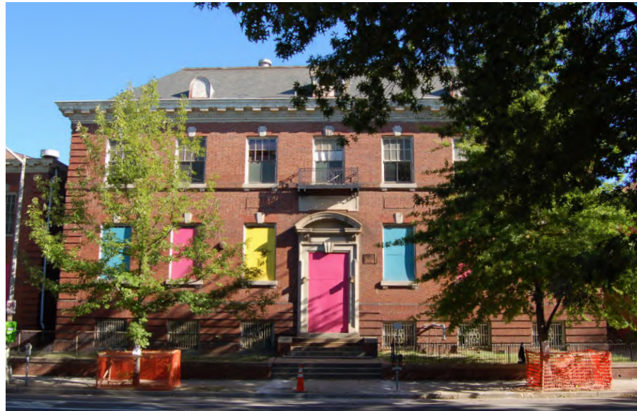
CENTRAL BUILDING - SOUTH ELEVATION (EXISTING CONDITIONS)
