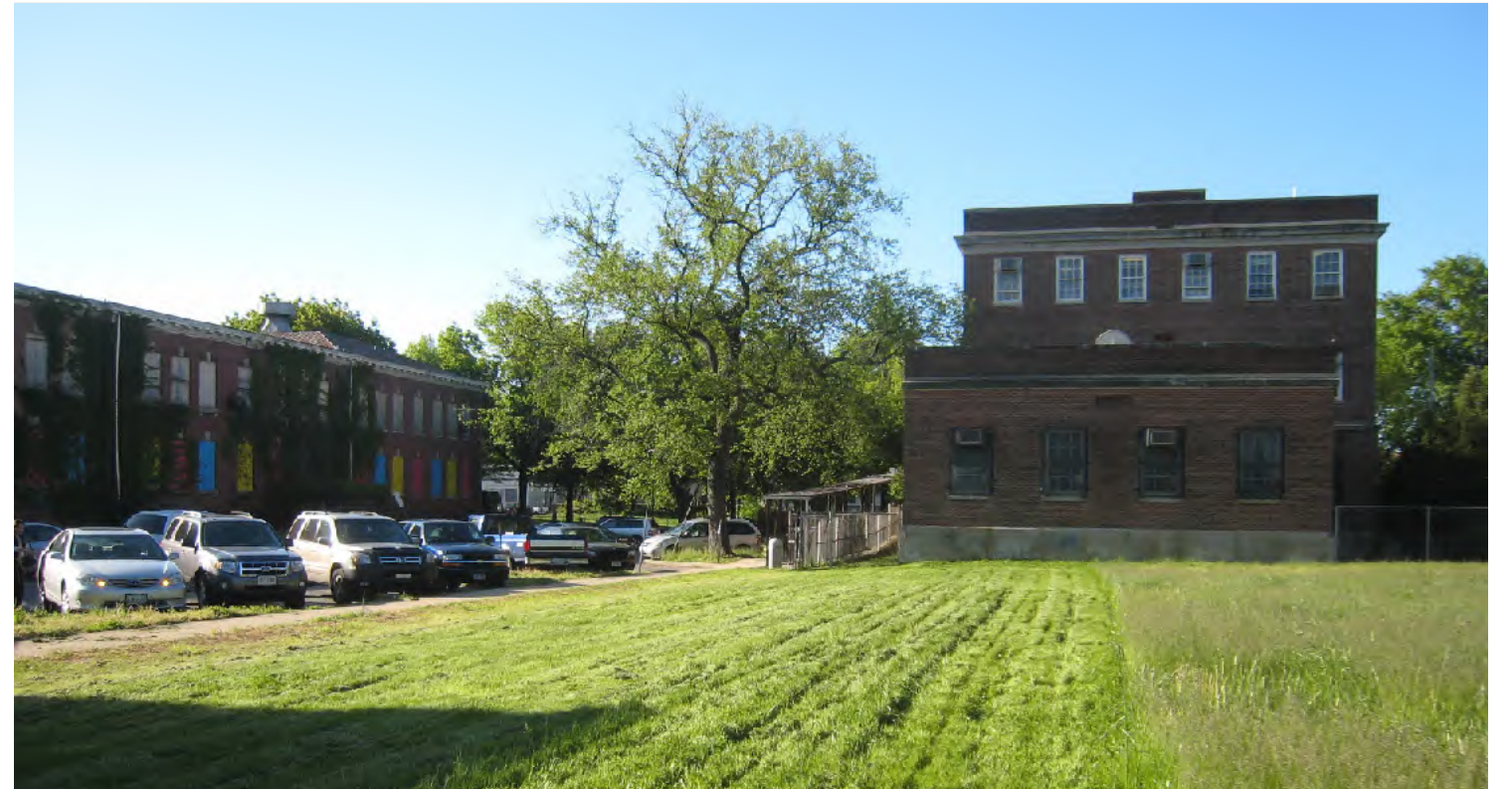
8 Corner of First Street & H Street looking southeast
